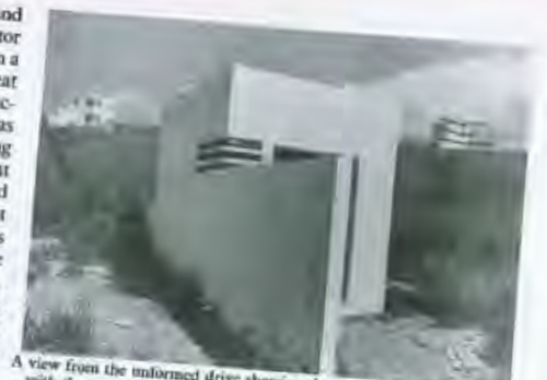
A view from the unformed drive showing the gate lodge and main house with the transformer house in the foreground. Later in the 'thirties, four houses by Basil Ward filled the space up to the lodge.
